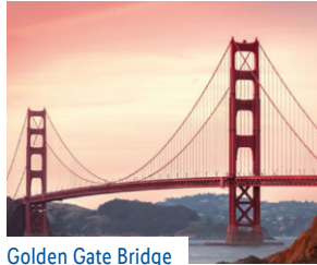
Golden Gate Bridge
