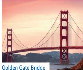
Golden Gate Bridge
